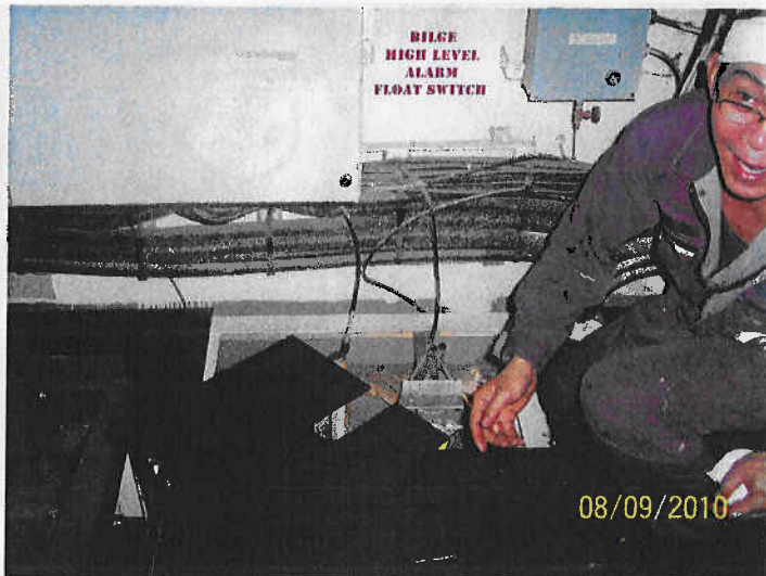
9/8/2010 20 Testing for'd bilge alarm.JPG
