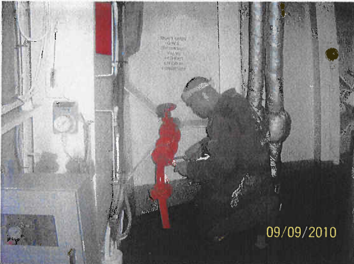
9/9/2010 10 Opening adjacent valve pipe for inspection.JPG
