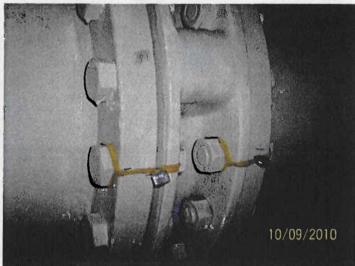
9/10/2010 07 ODME pumproom line flanges sealed.JPG
